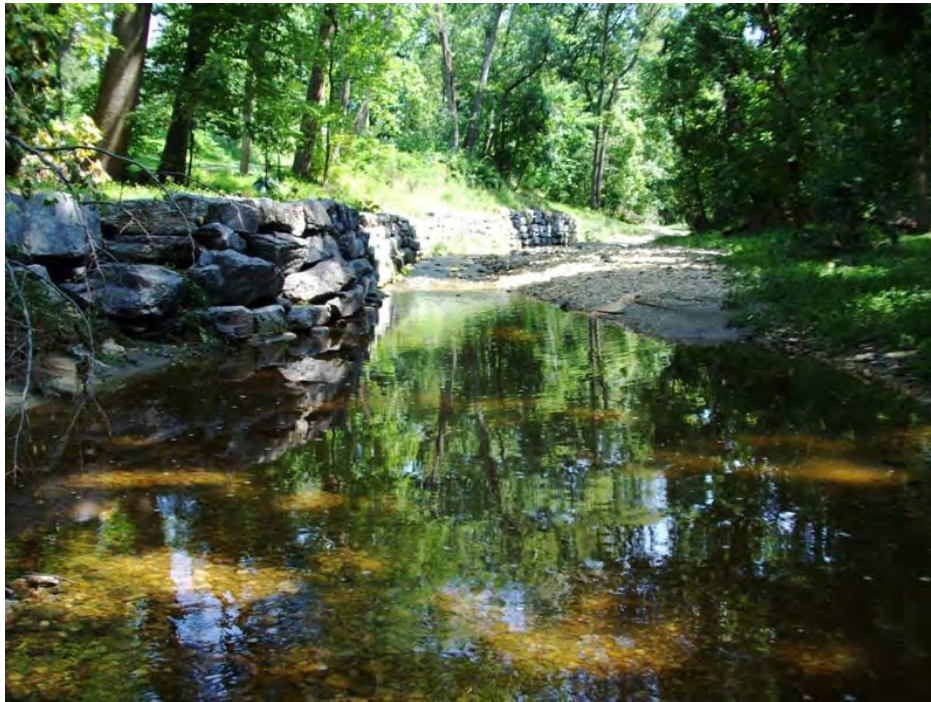
Figure 5. Photo of an Imbricated Riprap Wall.
