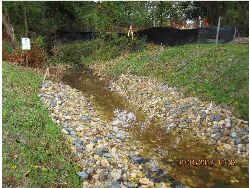
Figure 3. Photo of a Riffle Grade Control Structure.
