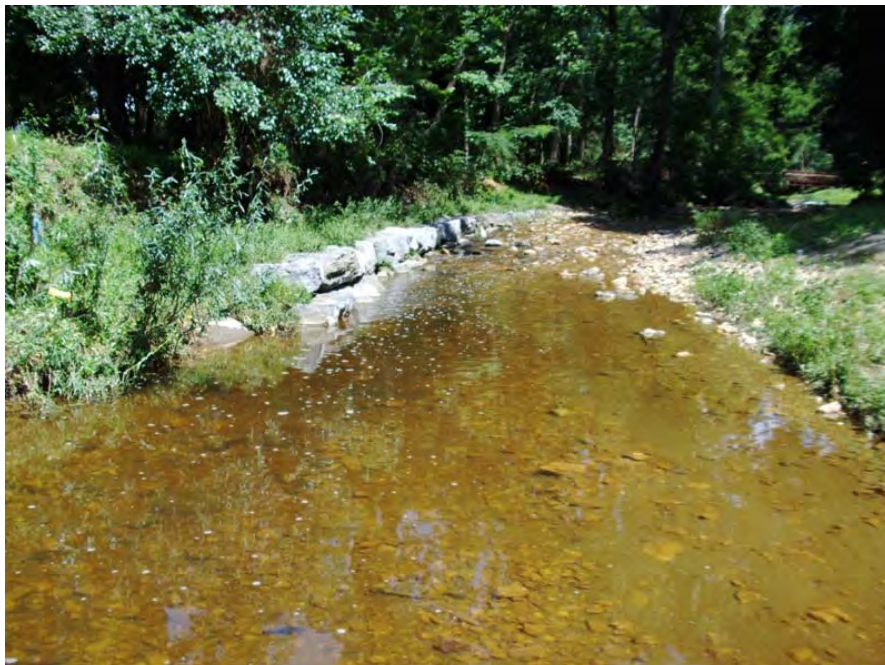
Figure 4. Photo of a Stone Toe Structure.
