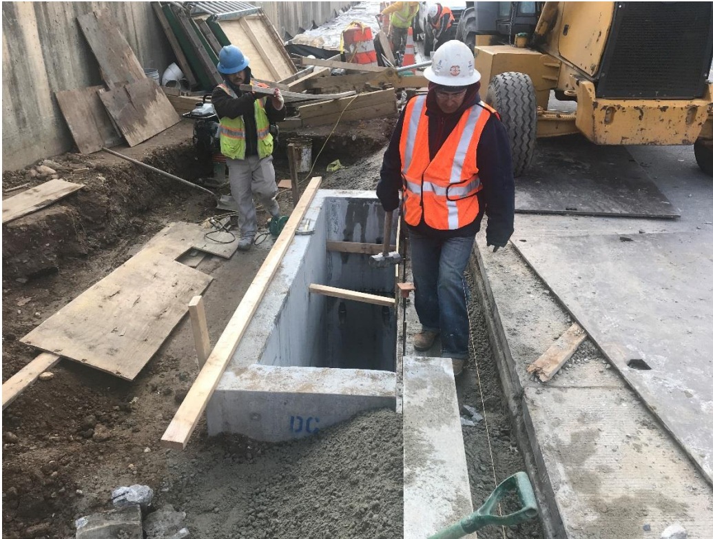
Inspected the newly reinstalled granite for the new catch basin on John McCormack
