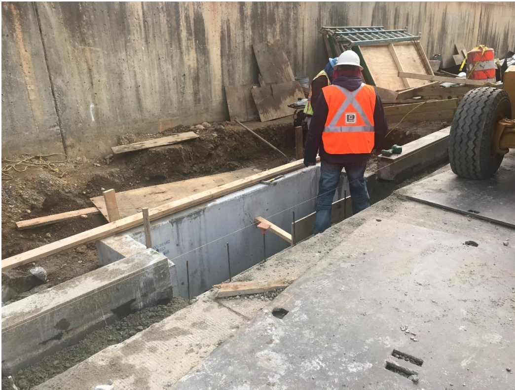
Preparing for the gutter installation at the new catch basin on new catch basin on John McCormack
