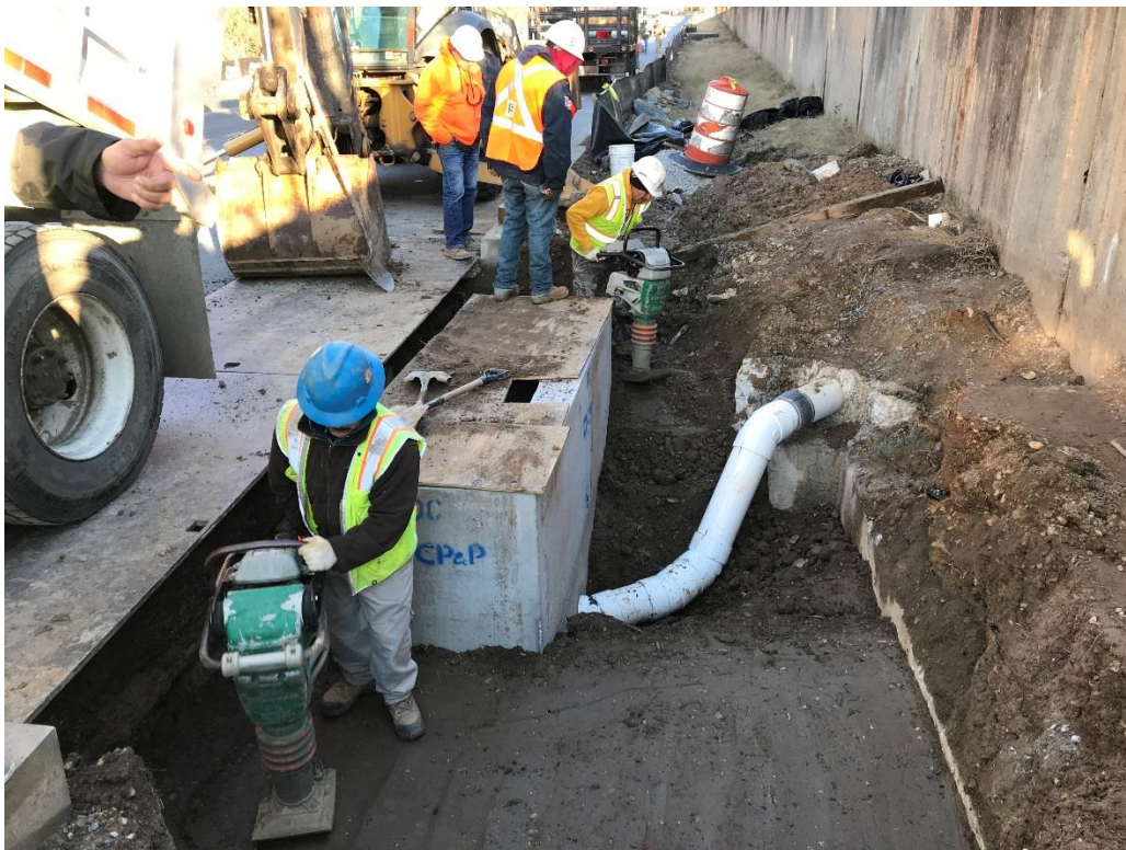
Backfilling the new catch basin on John McCormack
