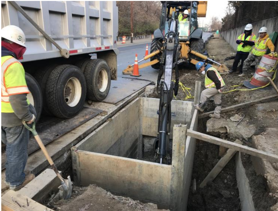
Preparing for the new catch basin installation on John McCormack
