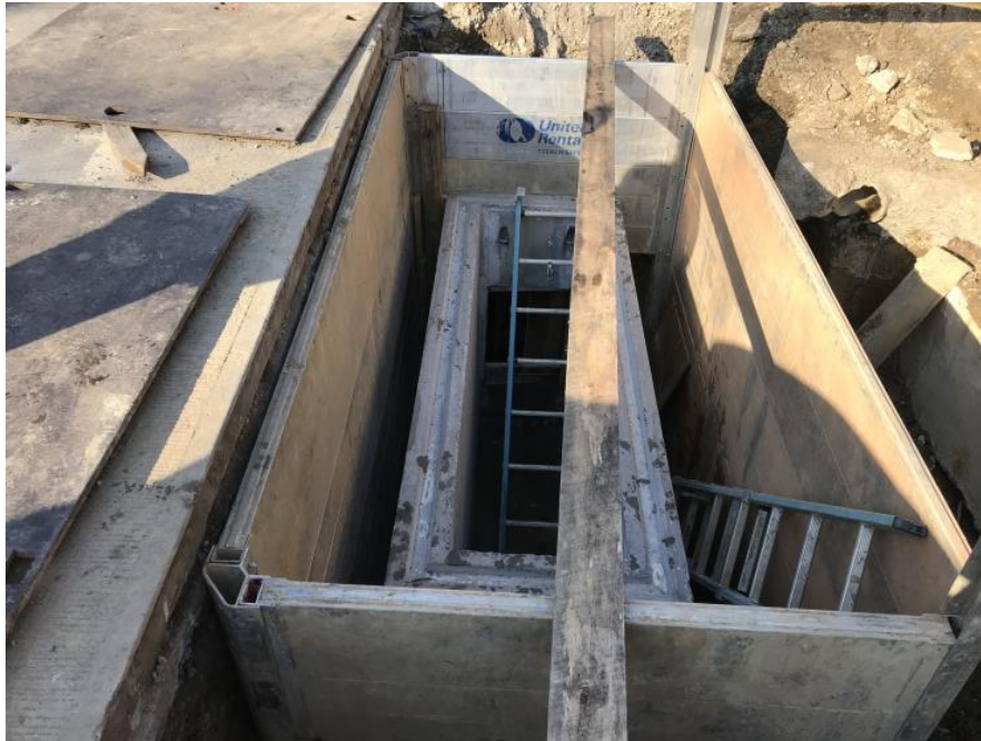
Installing the new catch basin on John McCormack
