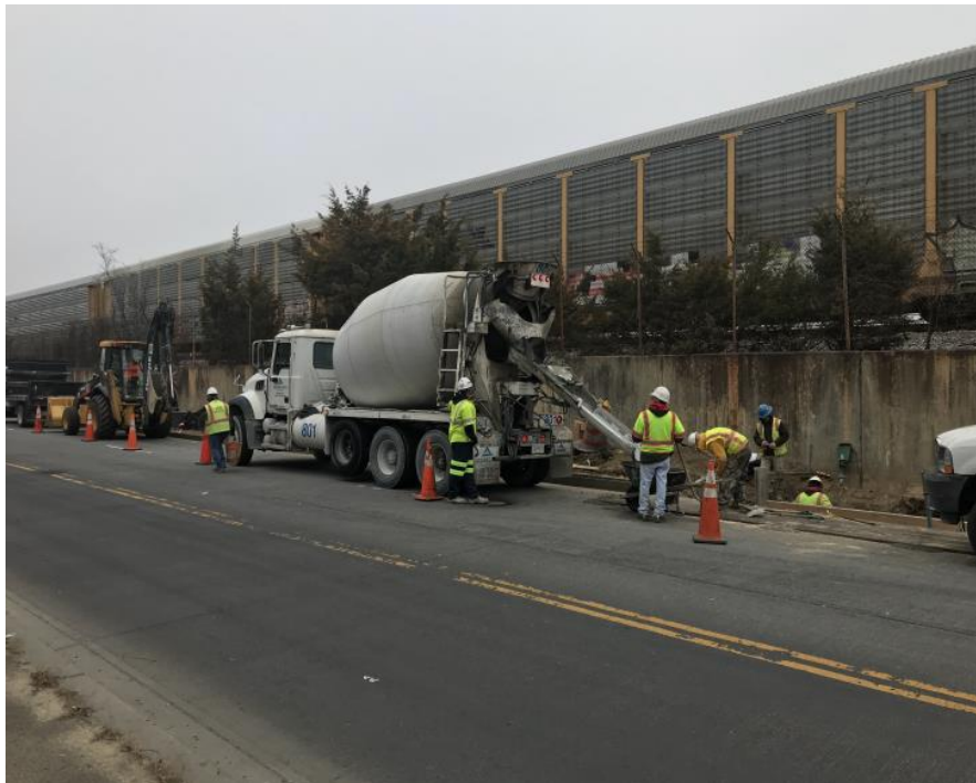
Pouring concrete around the pipe connection to the new catch basin on John McCormack
