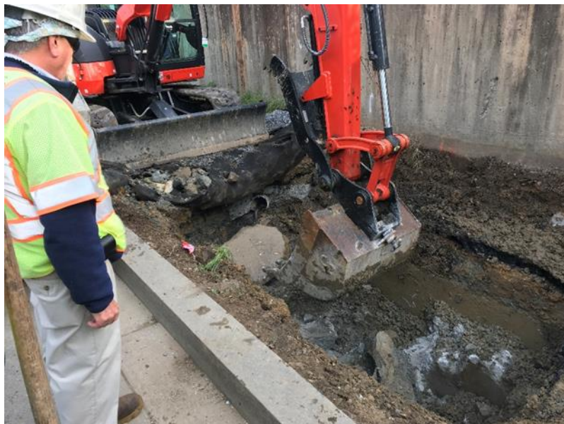
Excavation for the new catch basin near the South end of John McCormack
