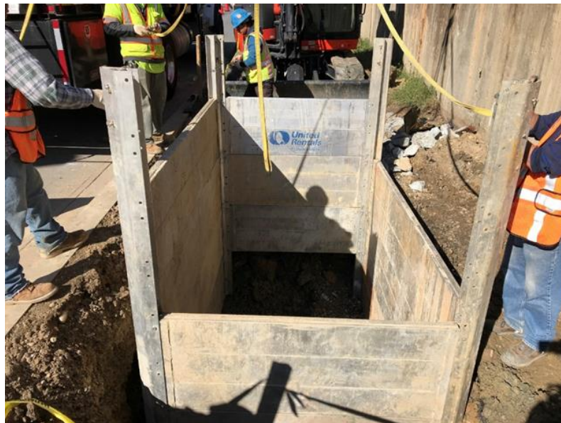
Excavation for new Catch Basin near the South end of John McCormack
