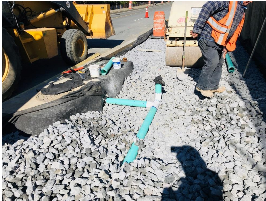
Underdrain Installation near the South end of John McCormack
