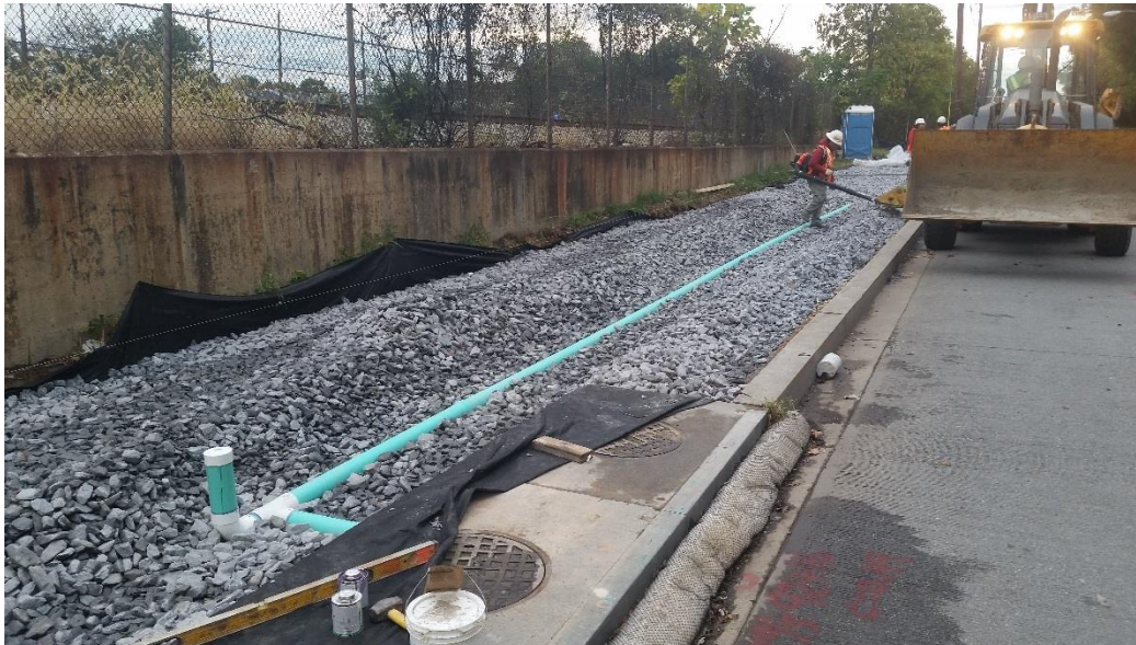
Underdrain Installation near the South end of John McCormack
