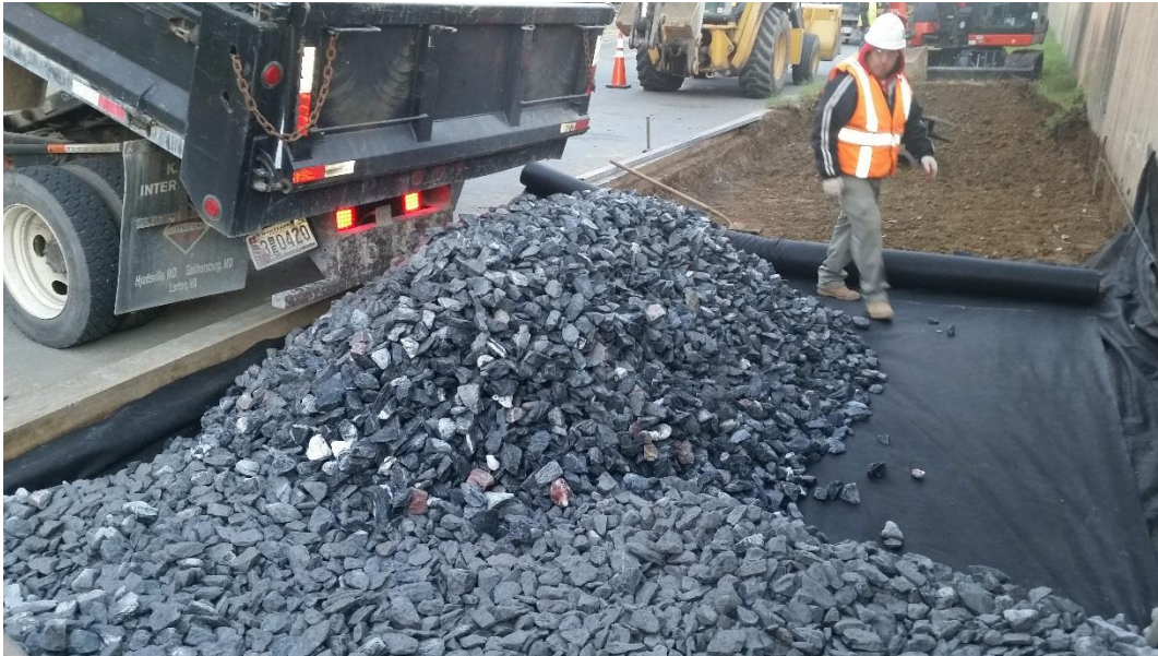
Placement of #2 stone near the South end of John McCormack
