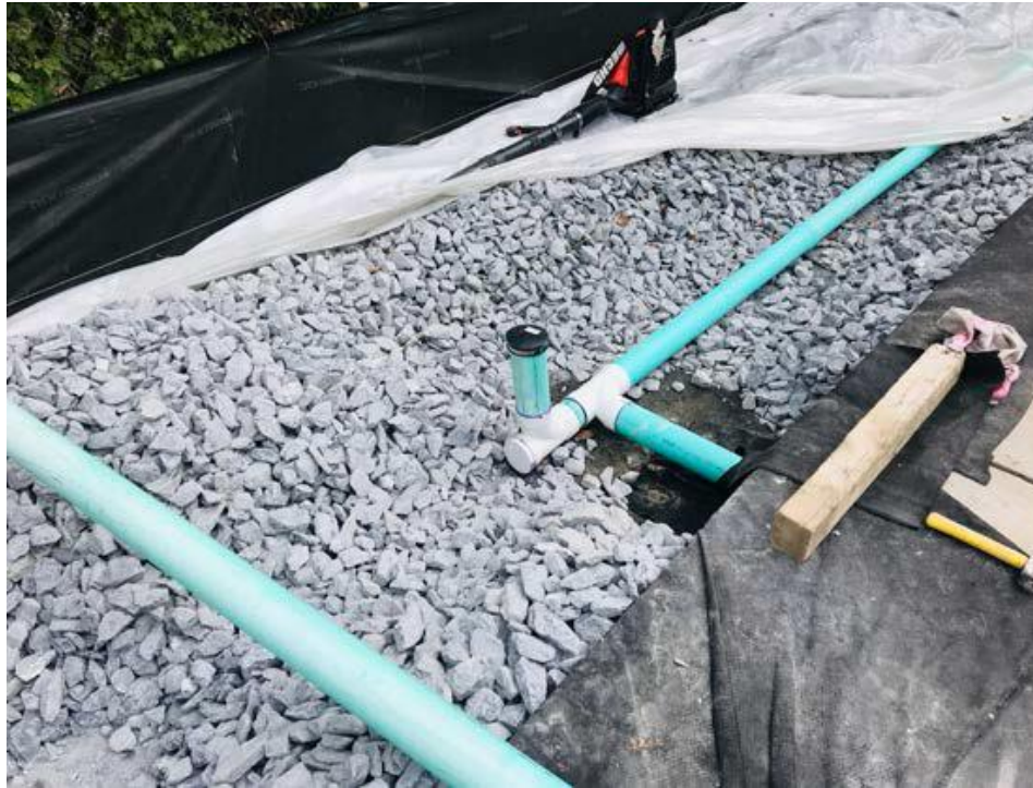
Underdrain Installation on the South end of John McCormack
