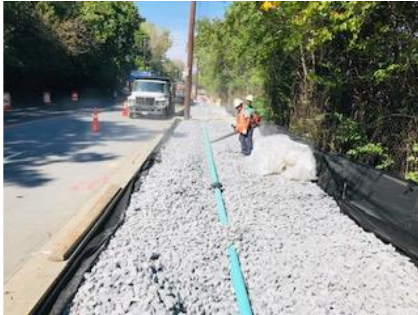
Underdrain Installation on the South end of John McCormack
