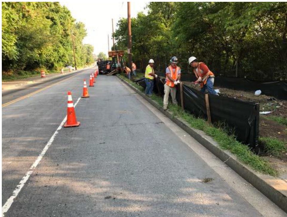
Installing Silt fence Near the South end of John McCormack
