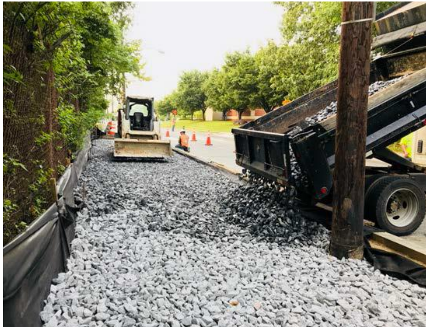
Placement of Number 2 Stone on the South end of John McCormack
