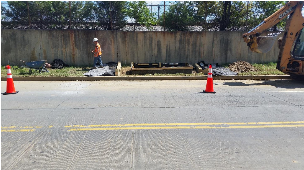
Installing Inlet protection around the double Catch Basin
