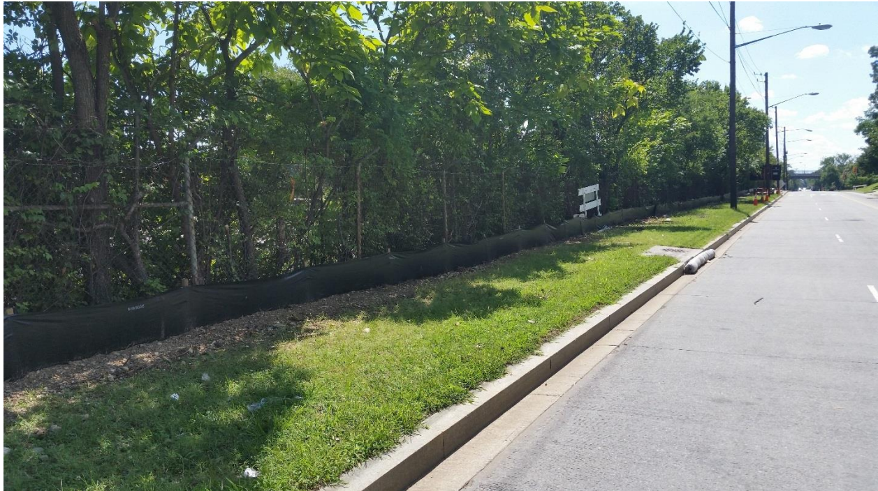
Silt Fence installed near the South End Of John McCormack
