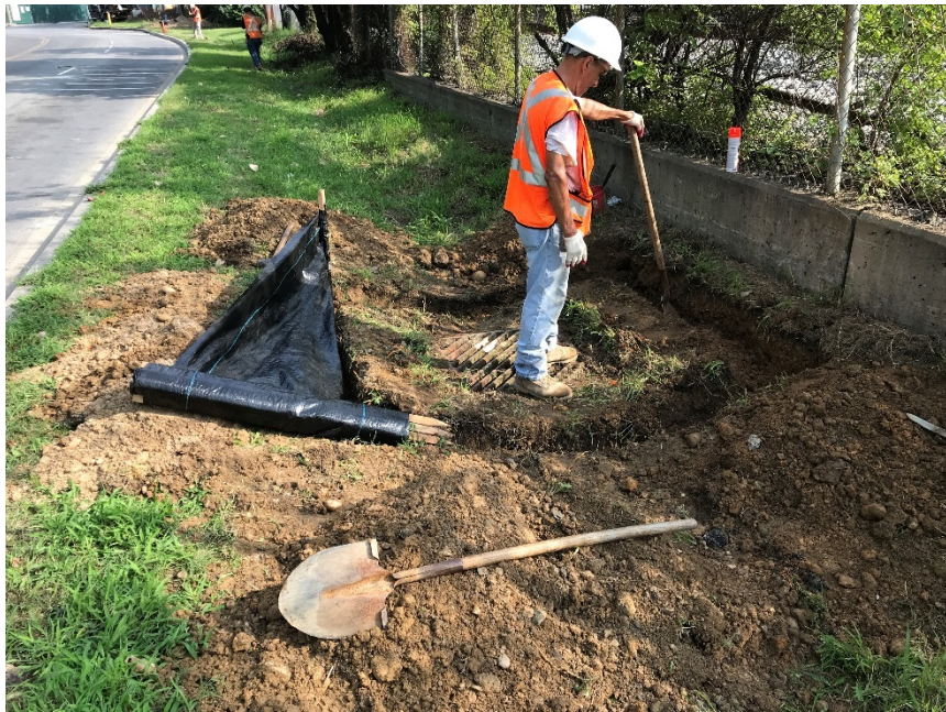
Installing Silt Fence around a Catch Basin
