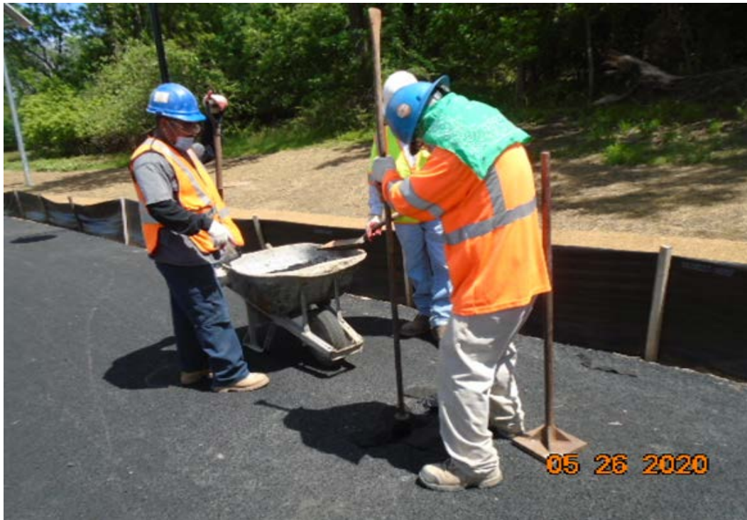
Phase B – Crew patching core hole at the trail
