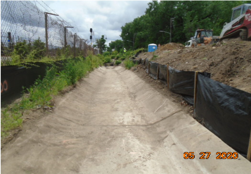
Phase D – Existing concrete ditch cleaned
