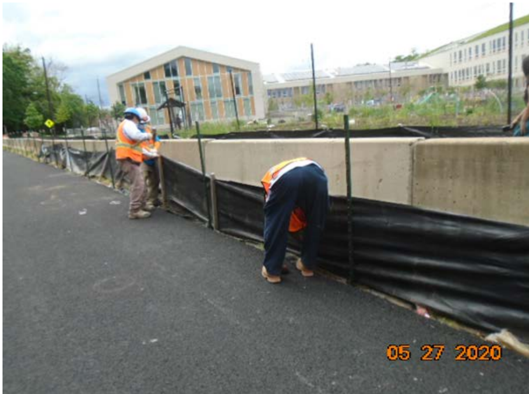
Phase B – Crew installing silt fence
