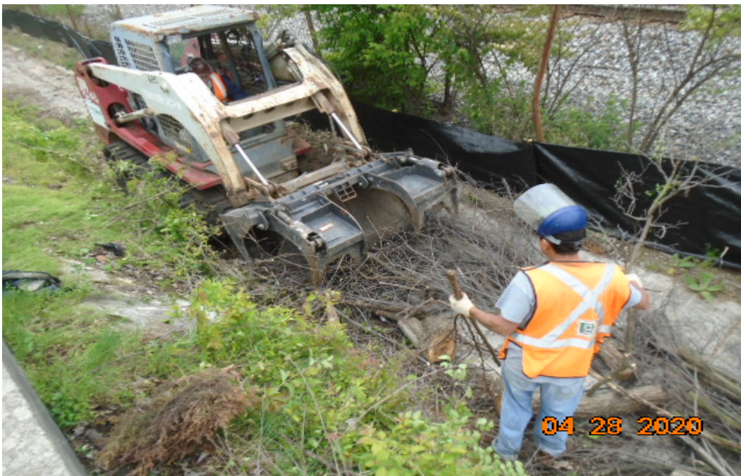
Phase D – Crew performing clearing and grubbing
