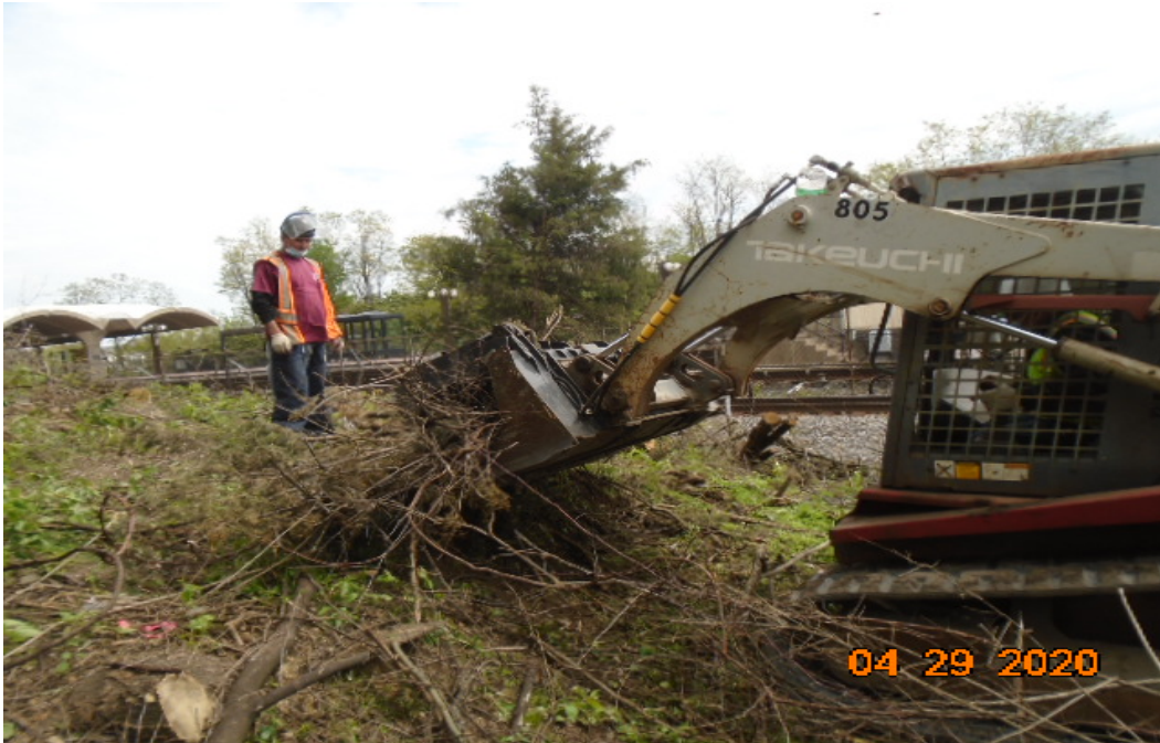
Phase D – Crew performing clearing and grubbing
