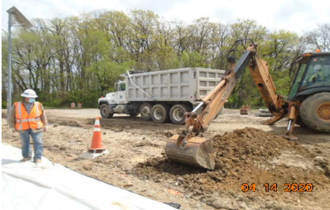
Phase B – Ditch construction along the South side on the trail
