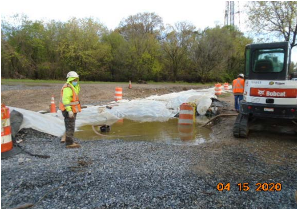
Phase B – Crew dewatering the project site due to the rainfall
