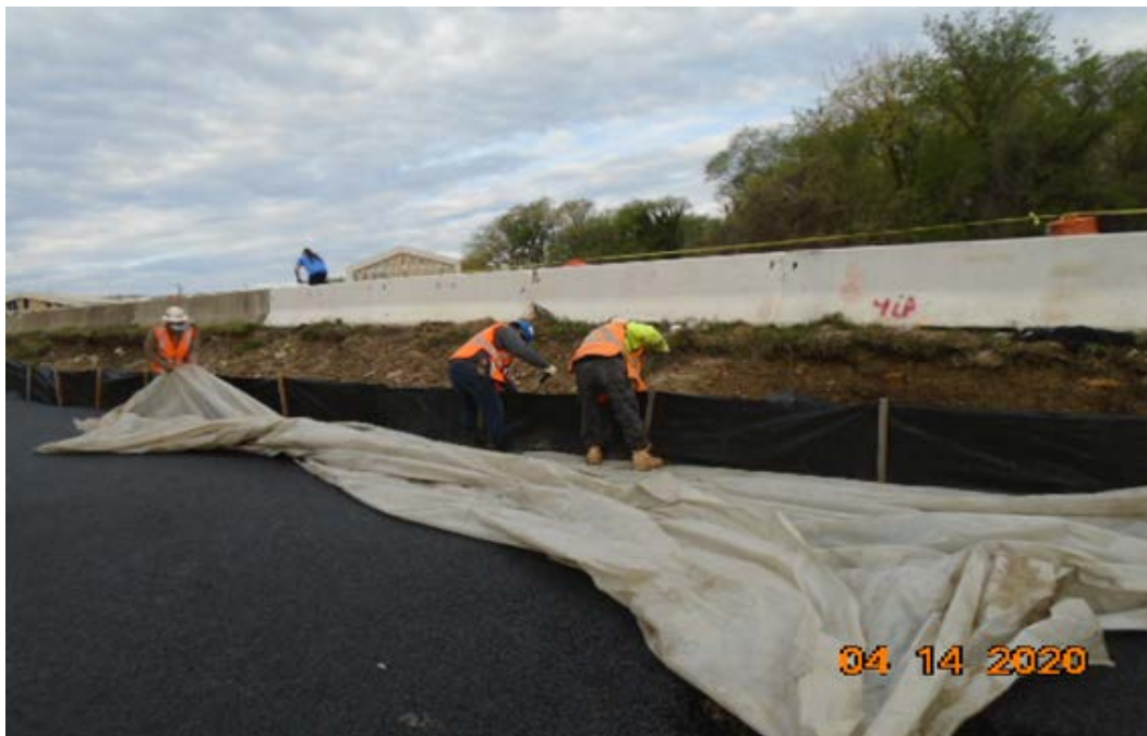
Phase B – Silt fence installation
