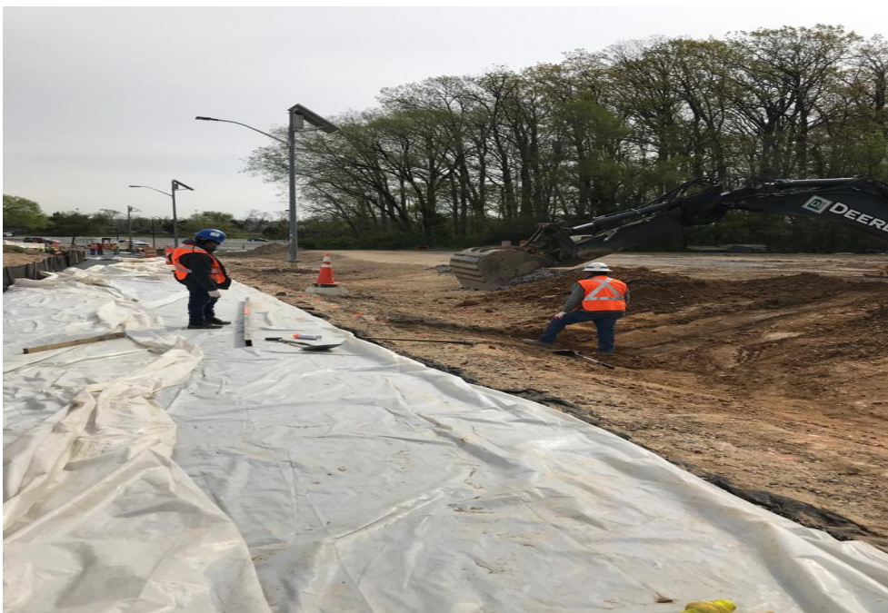
Phase B – Ditch grading along the North side of the trail
