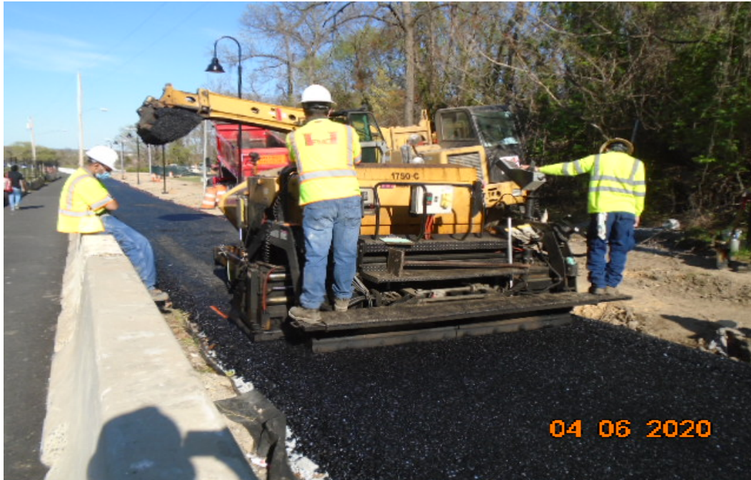
Phase B – Crew placing asphalt at the proposed trail
