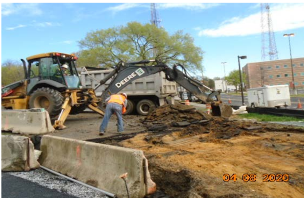
Phase B – Crew removing existing pedestrian trail
