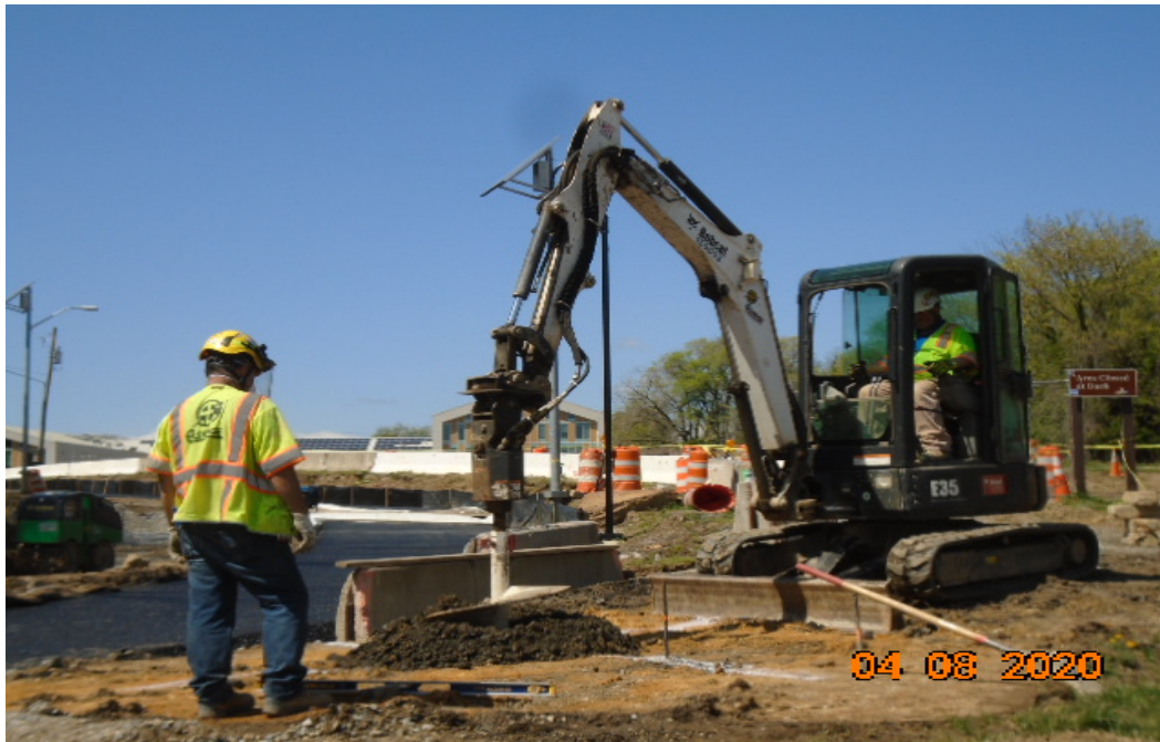
Phase B – Electrical crew preparing light pole foundation
