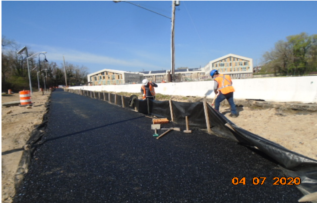
Phase B – Silt Fence Installation
