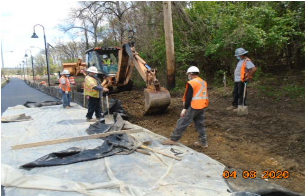
Phase B – Crew constructing the ditch along North side of the proposed trail
