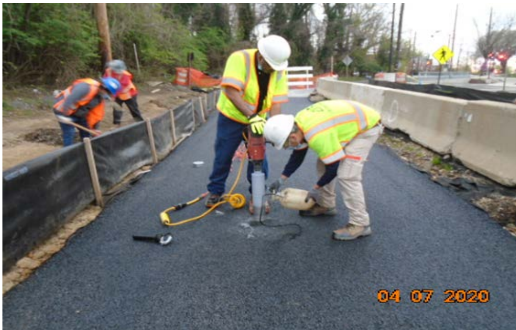
Phase B – Drilling of core asphalt at the proposed trail
