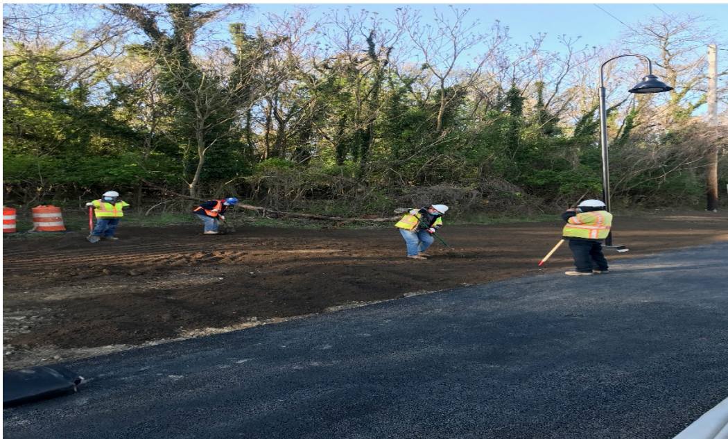
Phase B – Placing and grading of topsoil along the trail
