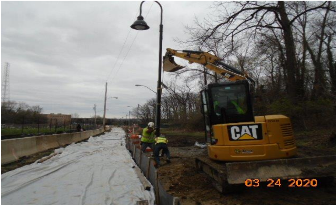
Phase B – Light Pole installation
