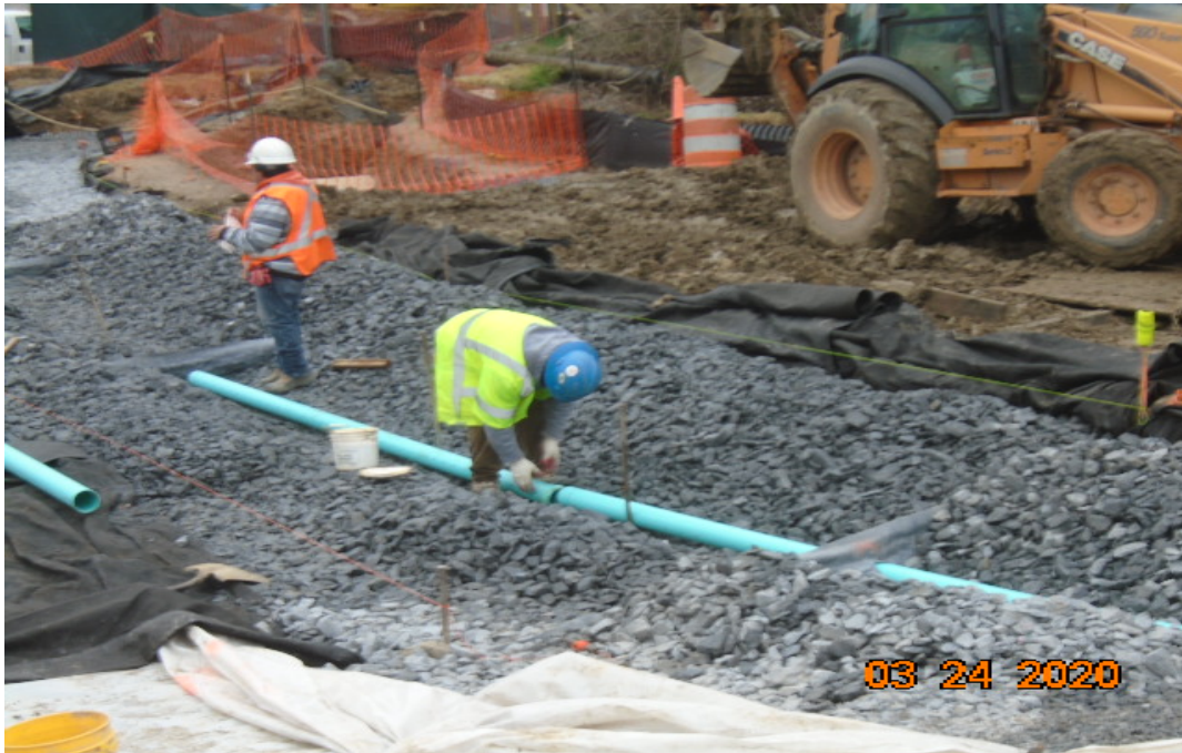
Phase B – Crew installing 4" underdrain pipes for the proposed trail
