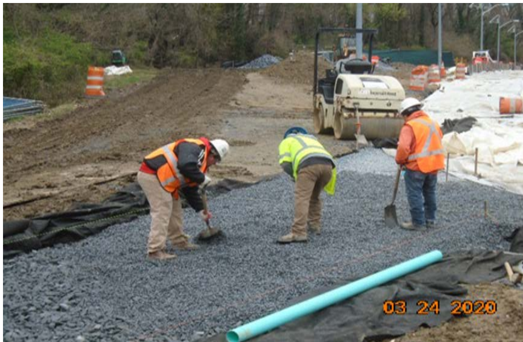
Phase B – Crew placing and grading stone at the proposed trail
