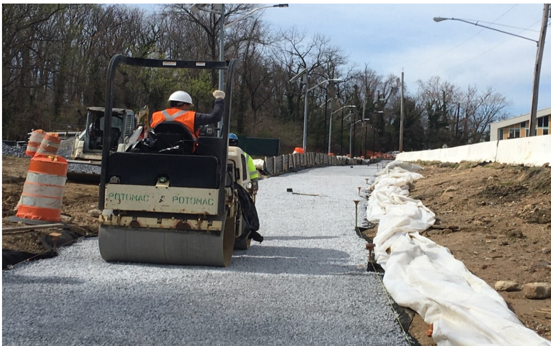
Phase B – Crew compacting the installed stone
