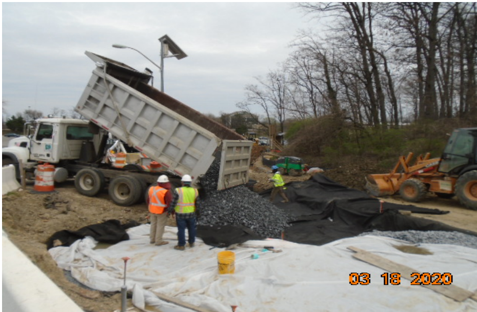
Phase B – Crew placing stone at proposed trench trail MBT 2-1
