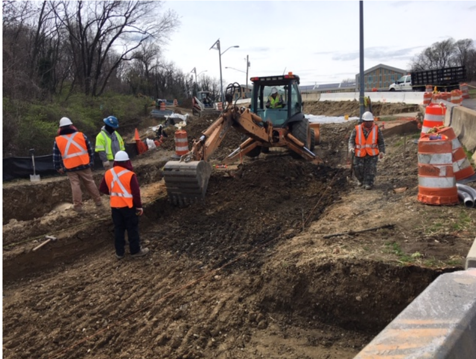
Phase B – Crew excavating the proposed trail trench
