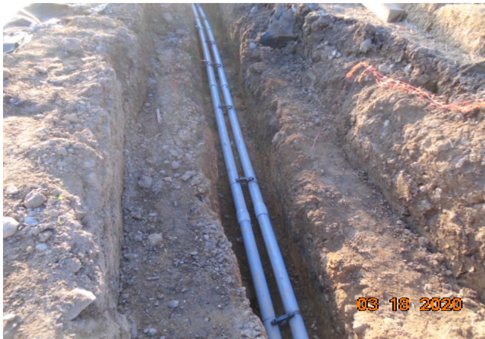
Phase B – Installed electrical line conduits
