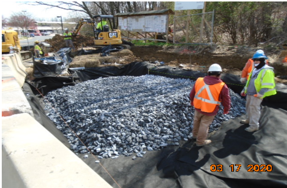
Phase B – Crew placing stone at MBT 2-1
