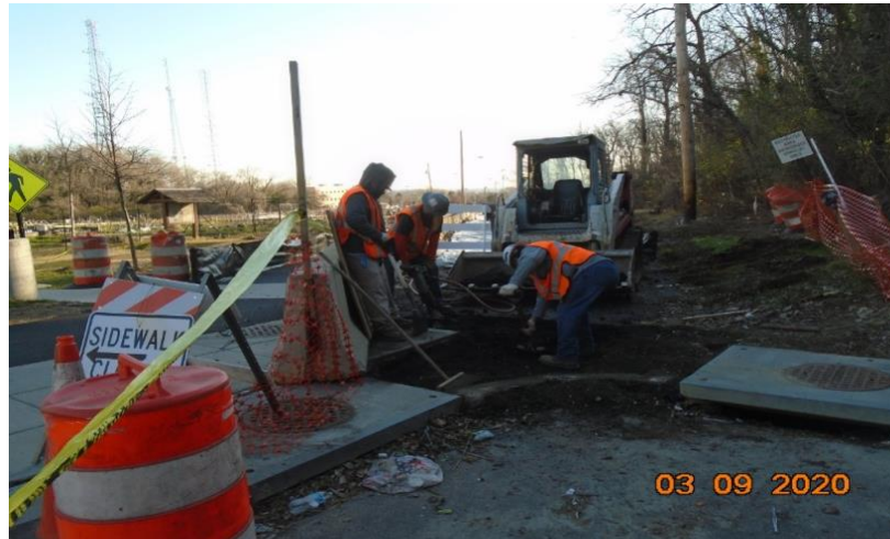
Phase B – removal of existing asphalt at Gallatin Street, N.E. and proposed street intersection
