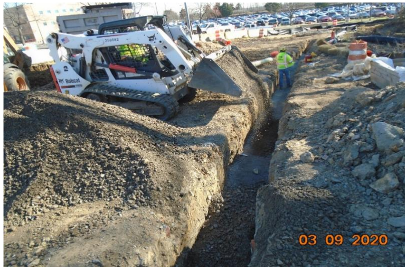
Phase B – Backfilling electrical trench MBT - 2
