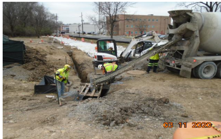
Phase B – Placing concrete at light pole foundation
