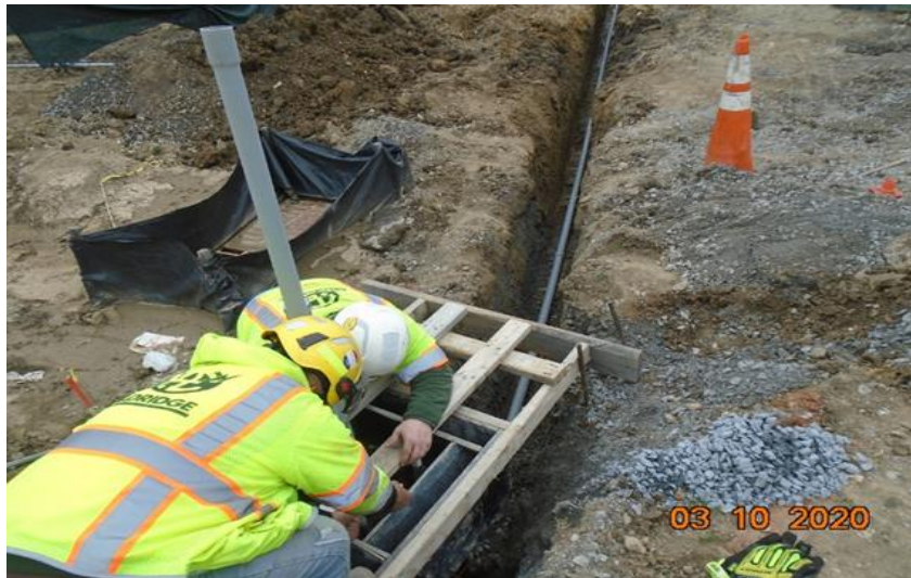
Phase B – Installing conduits at light pole foundation.
