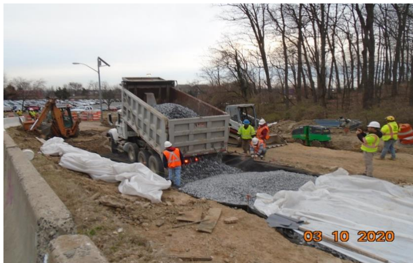
Phase B – Crew placing stone at MBT 2
