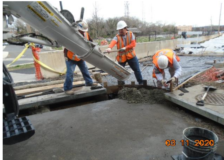
Phase B – Curb and Gutter concrete placement at the connection of Gallatin Street and the proposed trail
