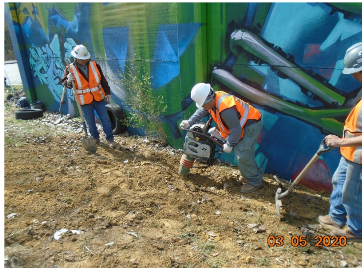
Phase D – Test pit hole backfill and compaction
