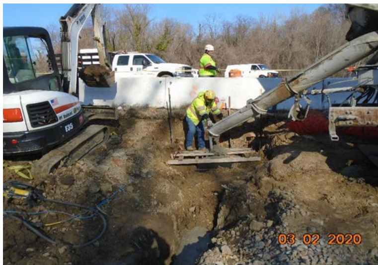
Phase B - Placing Concrete at Light pole Foundation MBT- 2
