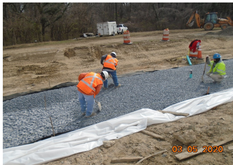
Phase B - Grading stone at MTB-2
