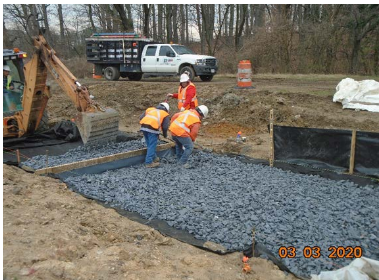
Phase B – Placing stone at MBT - 1
