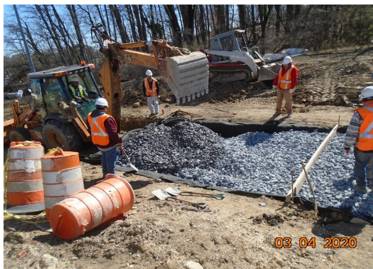
Phase B – Placing stone at MBT-2
