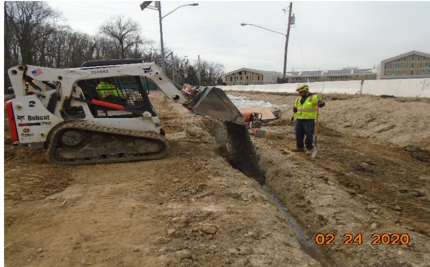
Phase B Crew backfilling the electrical Trench MBT- 2
