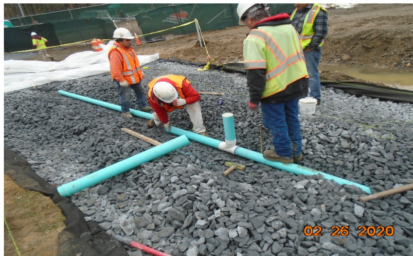
Phase B Crew Installing under drain pipe at MBT- 1
