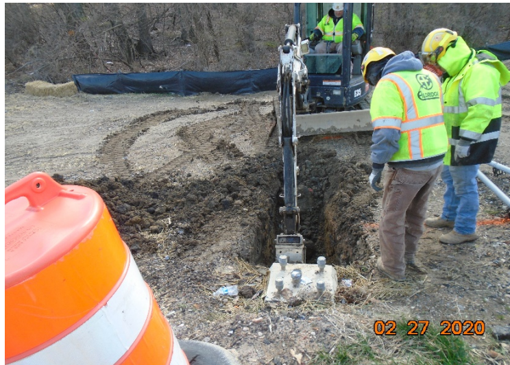
Phase B Excavating L3-PP Electrical Line
