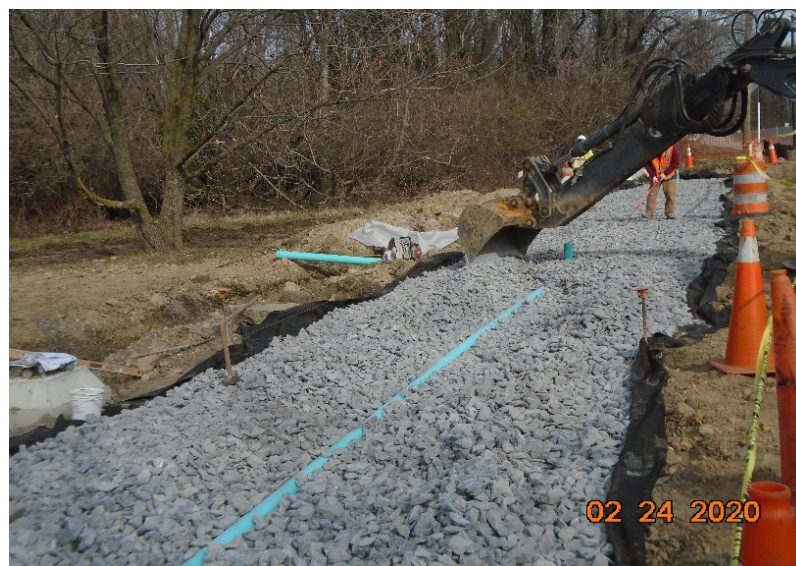
Phase B Installed 4" PVC Drain Pipe at MBT-1
