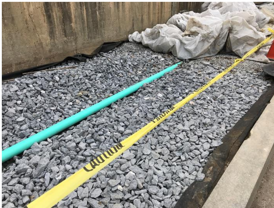
Underdrain near the new basin on John McCormack
