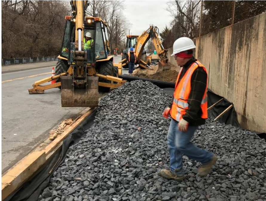
Stone placement near the new basin on John McCormack
