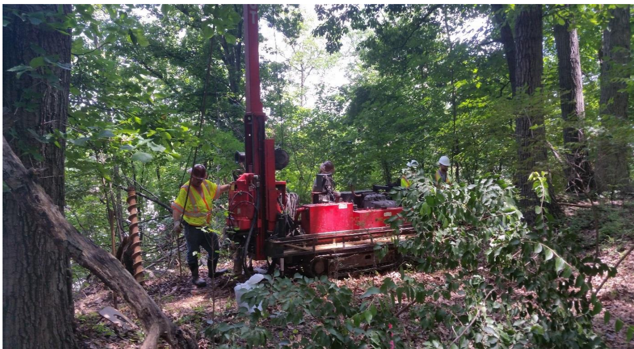
Structural Boring Phase D near First Place
