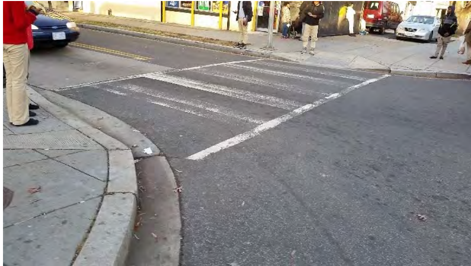
Figure 10 – Example of Worn Pavement Markings (at Randle Place)
