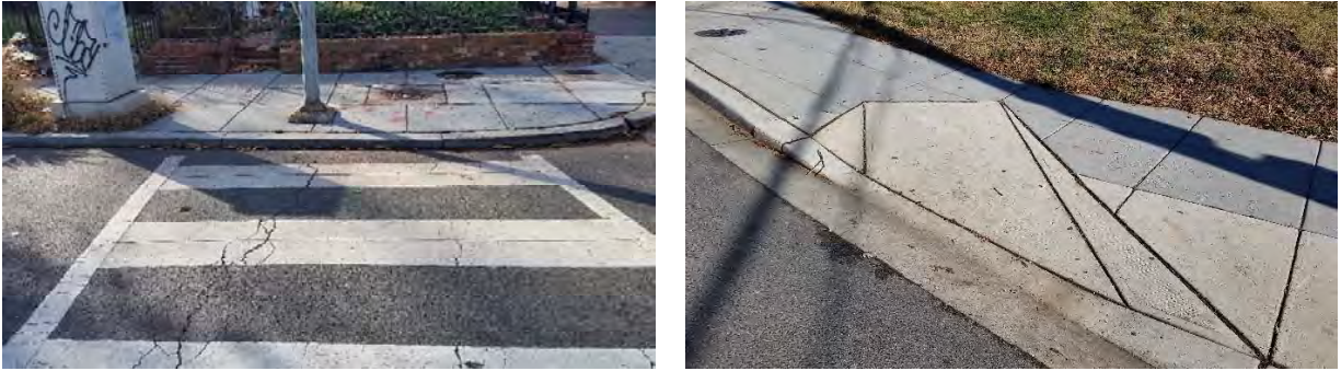
Figure 8 – Examples of Missing/Substandard ADA Ramps at Bruce Place (left) and Naylor Road (right)
