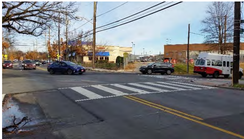
Figure 9 – Example of Utility Cut through Crosswalk (at 15 th Place)
