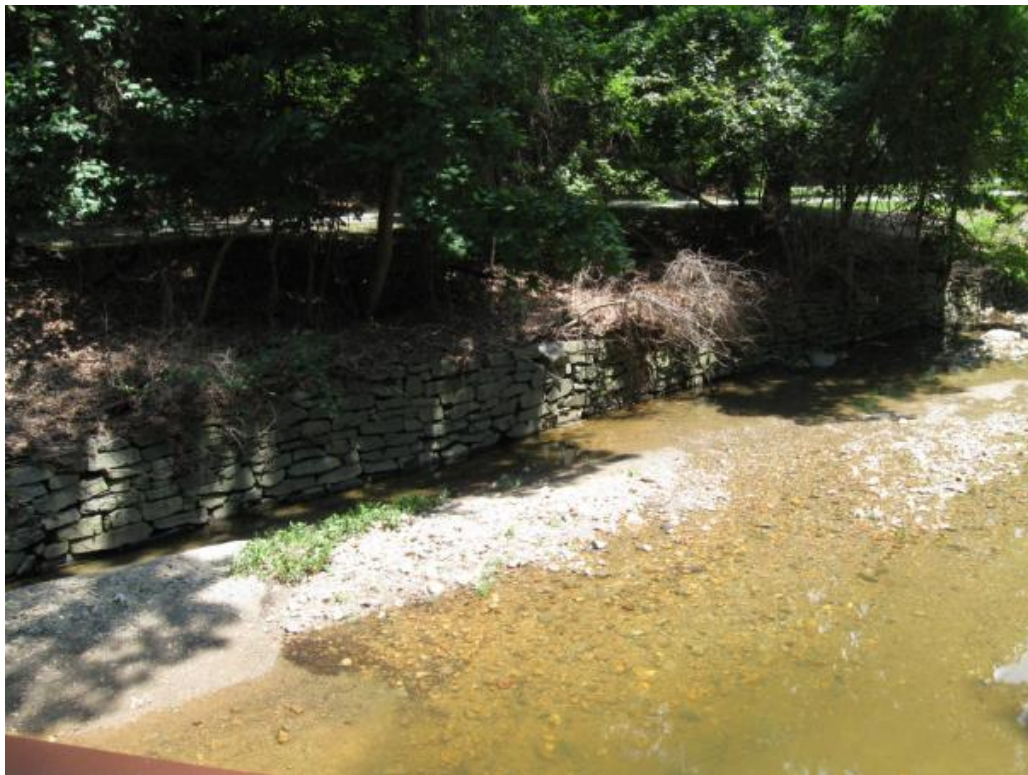
Figure 4. Dry laid tabular stone retaining wall (Segment 1) located on the east side of Broad Branch, between Broad Branch Road Bridge and Ridge Road Bridge.
