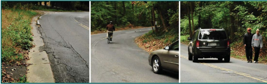
The existing roadway has deteriorated pavement and poor drainage and lacks safe means for bicyclists and pedestrians.
