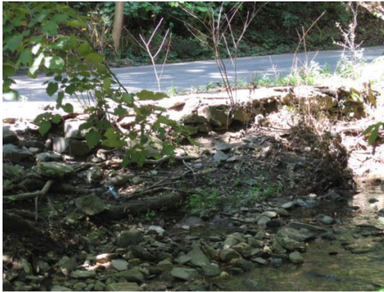
Figure 6. Dry laid stone retaining wall (Segment 3) located on the west side of Broad Branch, north of Soapstone Creek showing compromised stone blocks close to the road.
