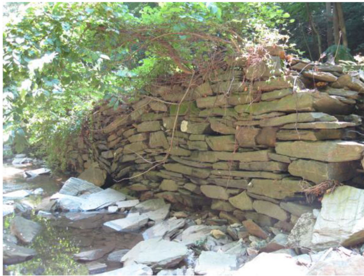
Figure 9. Dry laid tabular stone retaining wall (Segment 6) located on the west side of Broad Branch, north of Soapstone Creek.
