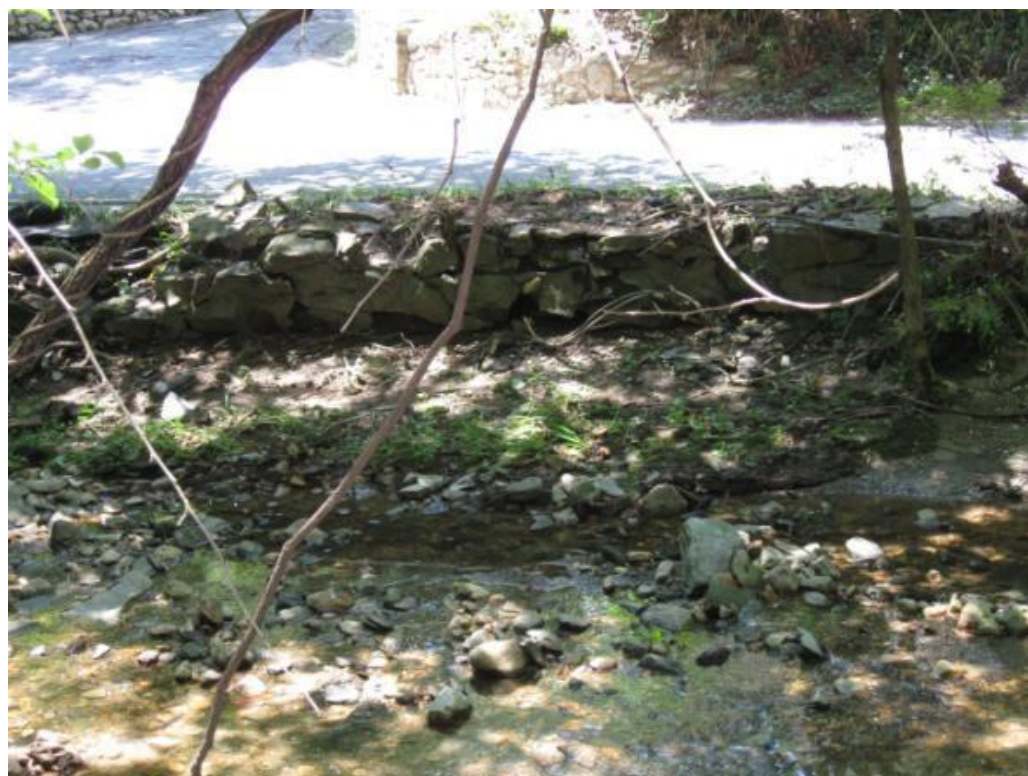
Figure 5. Dry laid stone retaining wall (Segment 2) located on the west side of Broad Branch, north of Soapstone Creek, showing a deteriorated wall of stone blocks, close to the road.
