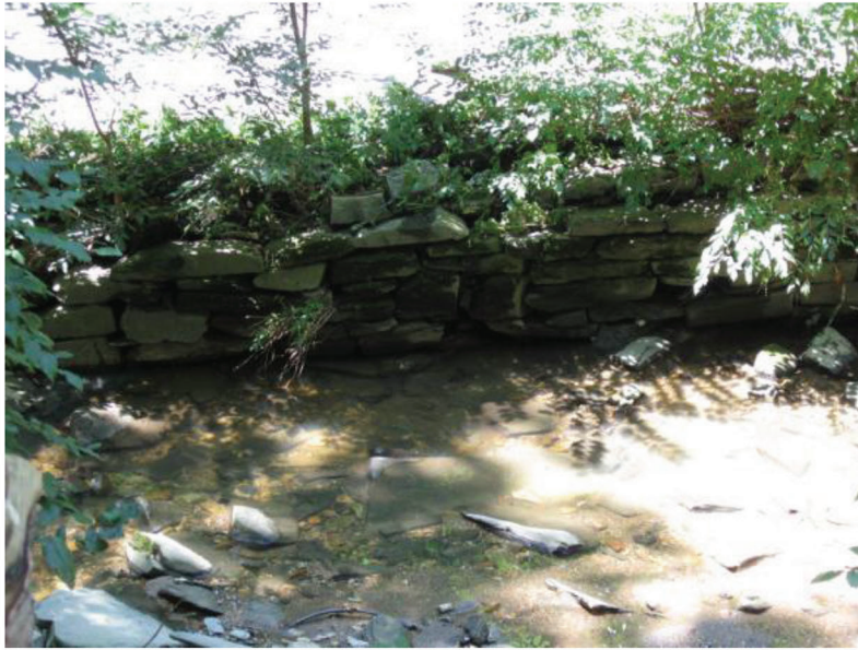
Figure 8. Dry laid tabular stone retaining wall (Segment 5) located on the west side of Broad Branch, north of Soapstone Creek.
