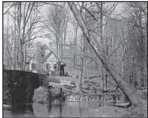
Figure 3-6. Pre-1934 Photograph of the Soapstone Creek Culvert (downstream side) without the wing walls. (E. B. Thompson, DC Public Library Photo Archives)
