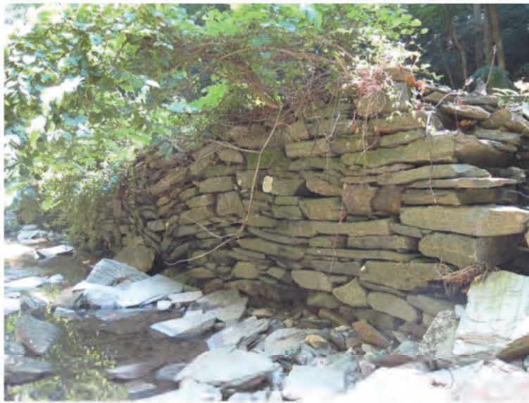
Figure 9. Dry laid tabular stone retaining wall (Segment 6) located on the west side of Broad Branch, north of Soapstone Creek.
