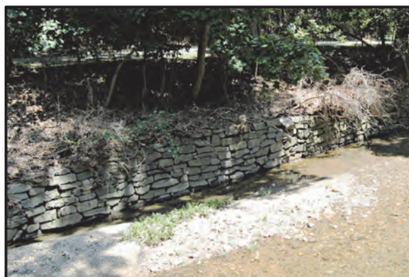
Figure 3-7. Dry laid rough cut stone in regular courses (large block) between the Broad Branch Road and Ridge Road Bridges
