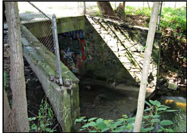
Figure 2-27. Concrete Box Culvert with Irregularly Coursed Stone Veneer on the north wingwall, looking northwest
