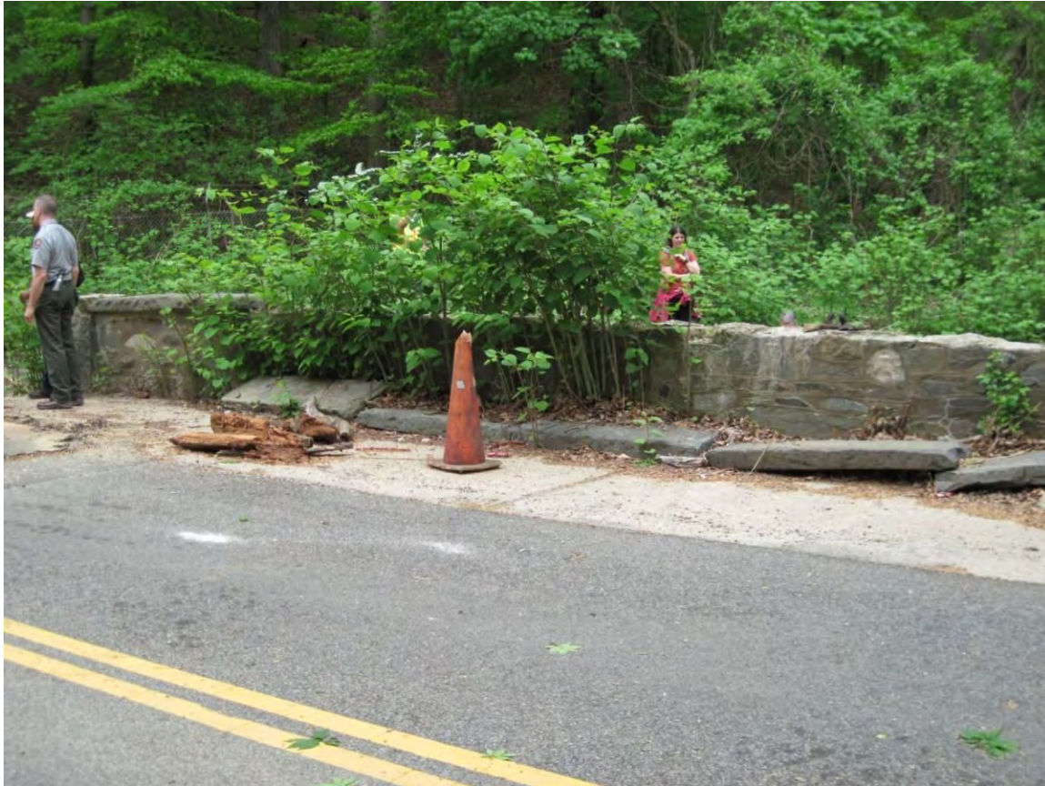
Figure 7. Roadside view of upstream headwall with original hand beveled capstone and beaded mortar joints (2011).
