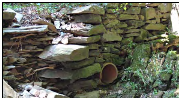
Figure 2-13. Storm Water Outfall with 18 inch diameter terra cotta pipe and stone retaining wall, west bank of Broad Branch Road
