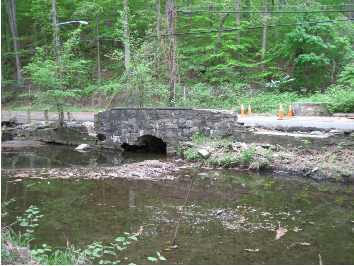
Figure 3. Downstream Headwall and Wing Walls of the Soapstone Creek Culvert at Broad Branch Run (2011).
