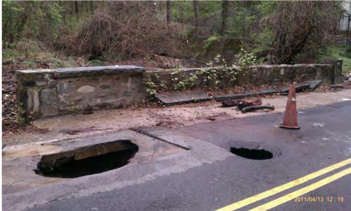
Figure 9. Holes created in the Broad Branch Road deck, looking upstream (2011).
