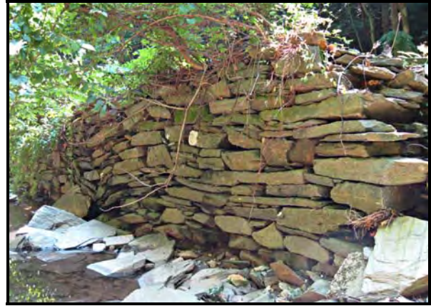
Figure 2-18. Dry laid rough cut stone in regular courses (combination of blocks and tabular pieces)
