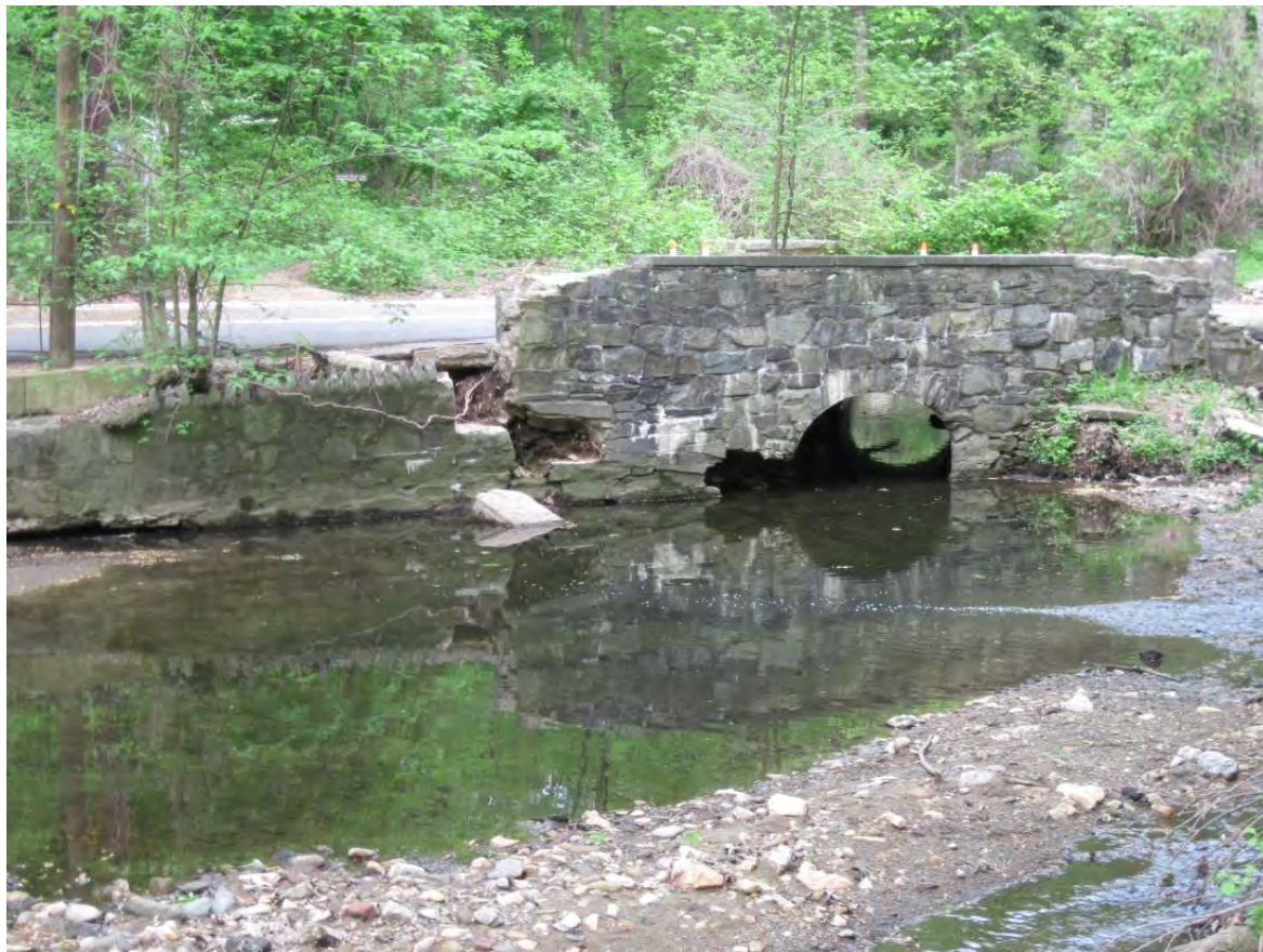
Figure 11. South Wing Wall and Downstream Headwall of Soapstone Creek Culvert after the collapse (2011).
