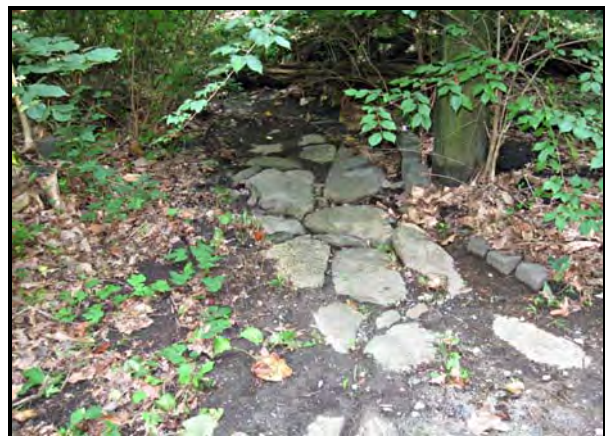
Figure 2-28. Example of Stone-lined Channel, located south of 27th Street between Broad Branch Road and Broad Branch
