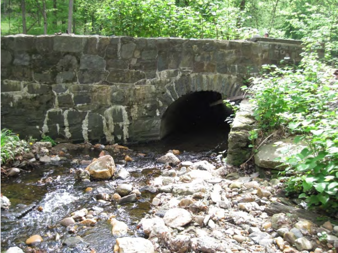
Figure 6. Upstream Headwall of Soapstone Creek Culvert and retaining wall (2011).
