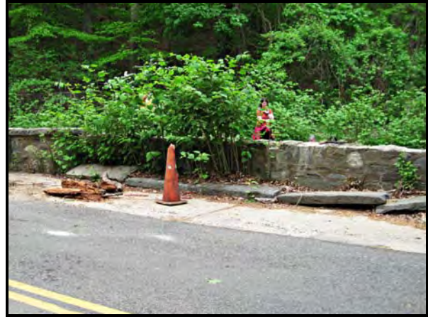
Figure 2-11. Roadside view of upstream headwall with original hand beveled capstone and beaded mortar joints
