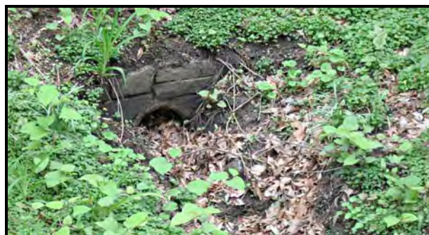
Figure 2-12. Storm Water Outfall with 15 inch diameter reinforced concrete pipe with regularly coursed rough cut stone headwall, west bank of Broad Branch, north of Ridge Road
