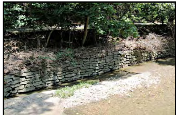
Figure 2-17. Dry laid rough cut stone in regular courses (large block) between the Broad Branch Road and Ridge Road Bridges
