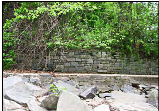
Figure 2-16. Mortared Ashlar Stone Wall with concrete spillway south of Broad Branch Road Bridge
