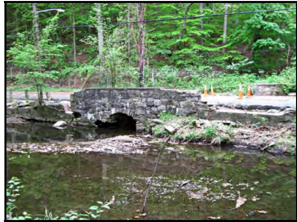
Figure 2-8. Downstream Headwall and Wing Walls of the Soapstone Creek Culvert at Broad Branch (2011)
