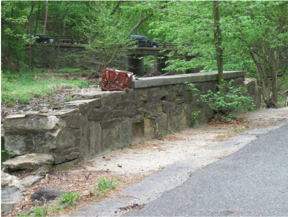
Figure 5. Roadside view of the downstream headwall with machine cut capstones, with Ridge Road Bridge in the background (2011).
