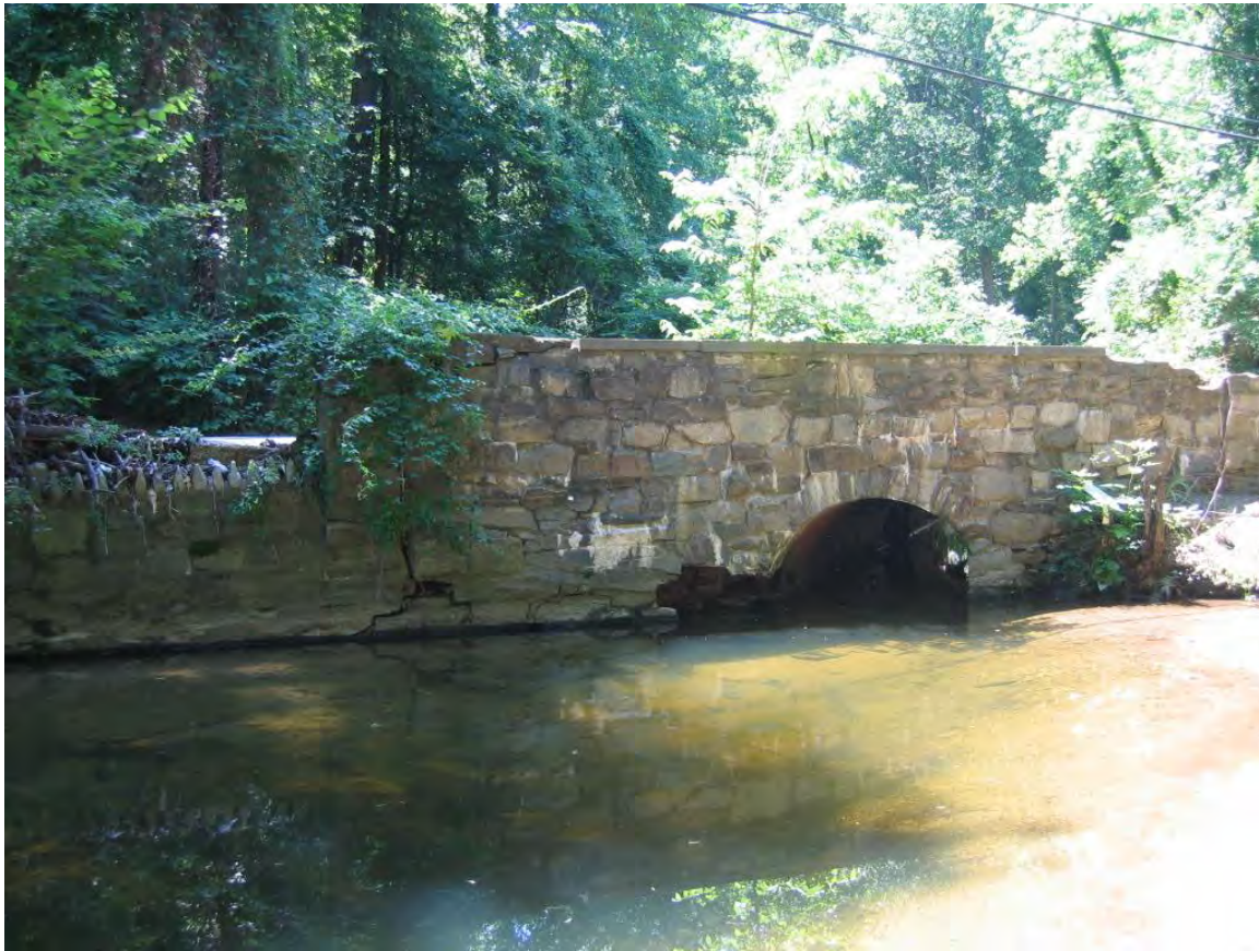
Figure 10. South Wing Wall and Downstream Headwall of Soapstone Creek Culvert pre-collapse (2009).
