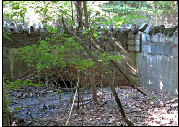
Figure 2-26. Storm Water Inlet with 36 inch diameter reinforced concrete pipe surrounded by brick and concrete with crenellated stone headwall and wingwall
