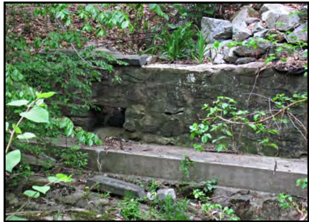
Figure 2-24. Irregularly coursed rough cut stone retaining wall on east side of 27 th Street Bridge
