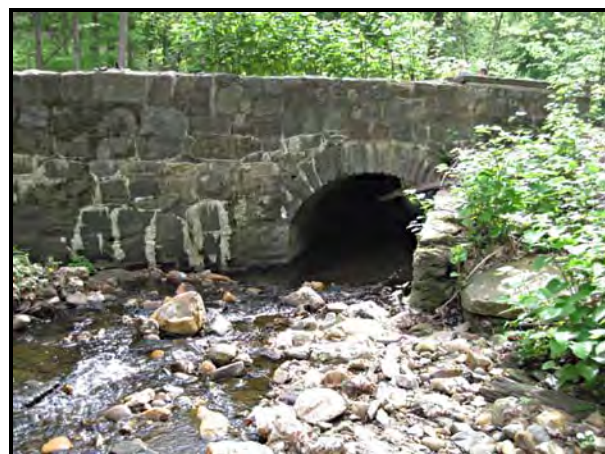
Figure 2-10. Upstream Headwall of Soapstone Creek Culvert and Retaining Wall
