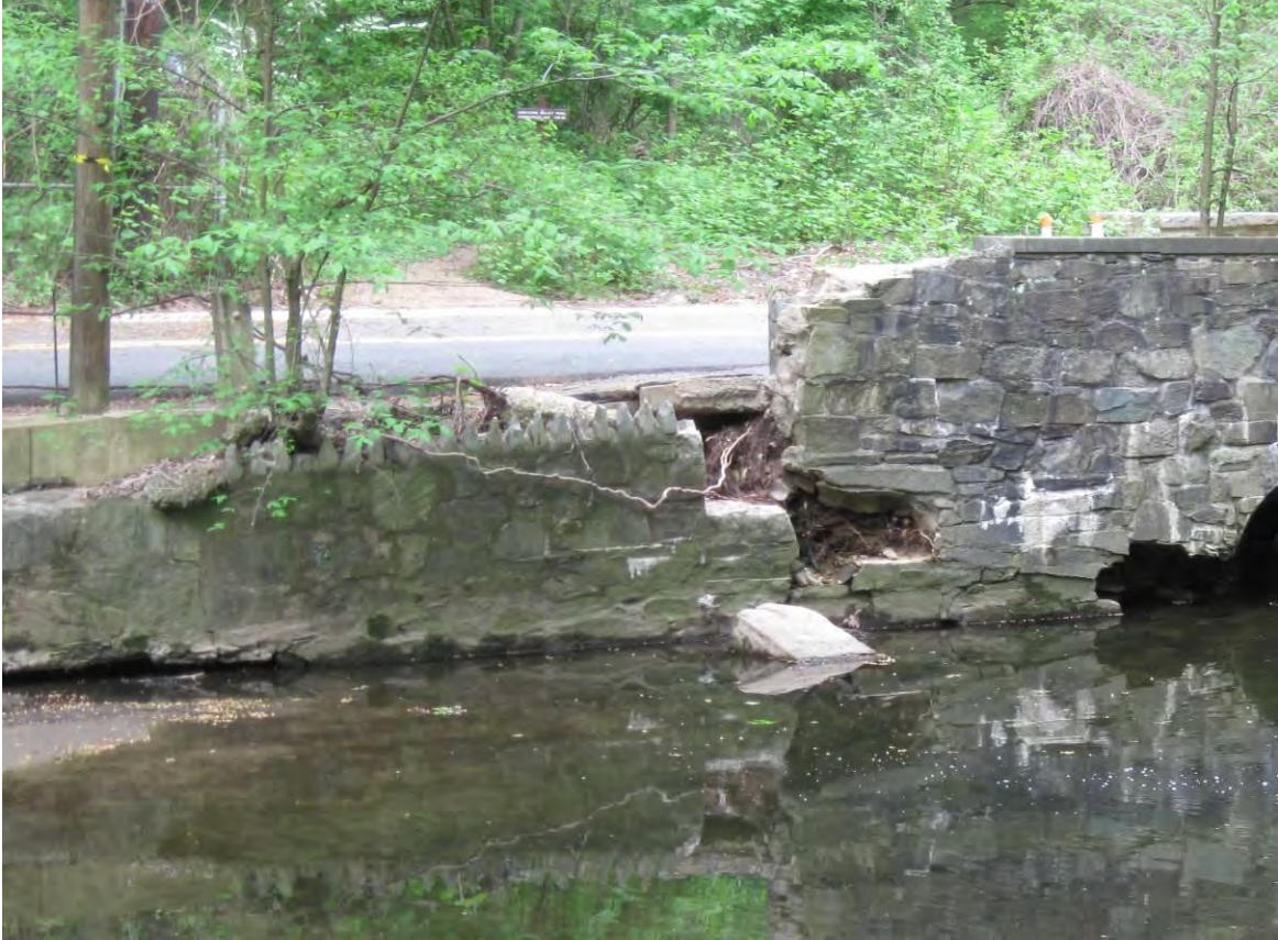
Figure 4. South Wing Wall of Soapstone Creek Culvert with Crenellated Treatment (2011).
