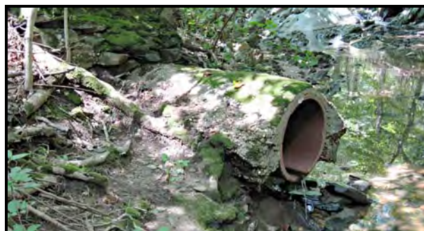
Figure 2-14. Storm Water Outfall with 24 inch diameter vitrified clay pipe, stone headwall, and concrete repair, west bank of Broad Branch, south of Brandywine Avenue
