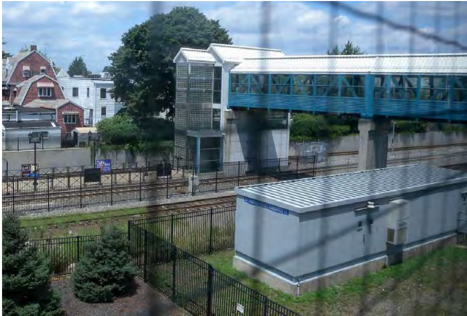
Figure 2-19: TPSS design to complement a mixed-use area
